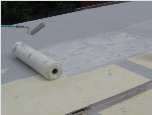
Glass fibre mat laid into wet bodycoat
