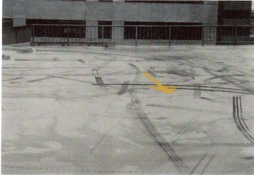
FIGURE 1: Upper Deck, Willis Street Carpark
