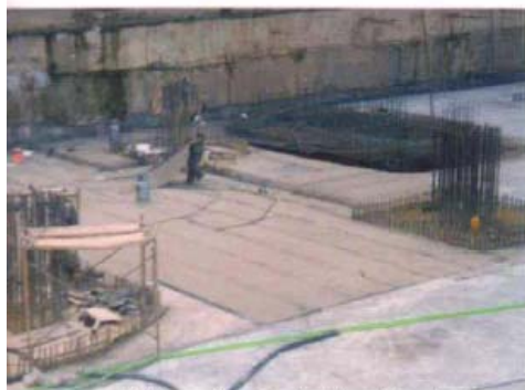
Waterproofing Park Hyatt hotel, Hanoi - Vietnam
