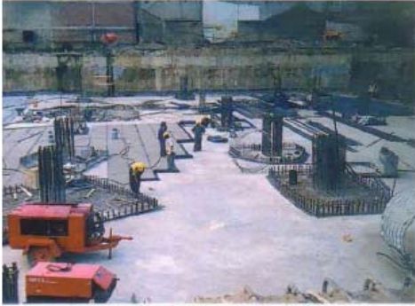
Waterproofing of basement with pilar caps and beams
