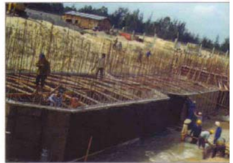
Waterproofing ceramic factory, Da Nang - Vietnam
