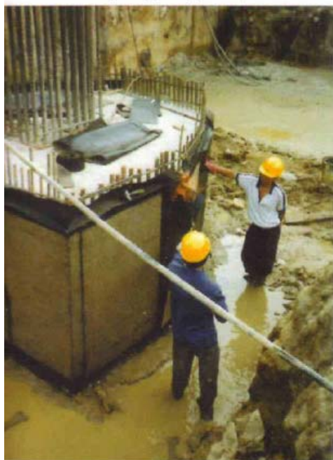
Waterproofing Park Hyatt hotel, Hanoi - Vietnam
