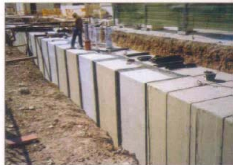
Waterproofing of utility tunnel, Valencia - Spain
